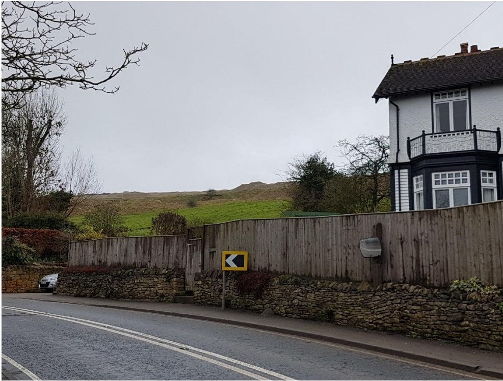
End of Cleeve Hill Settlement – above the B4632 - Hilcrest
